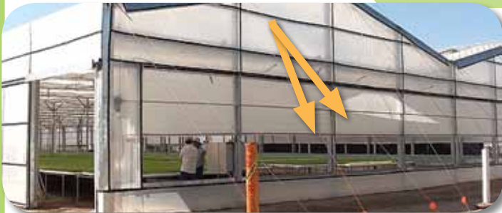
External cable bracing on the gable ends
