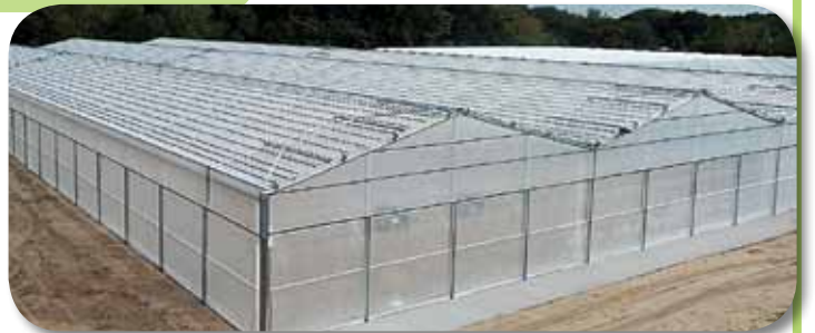
Roof purlins eliminate gable cable bracing ( optional upgrade )
