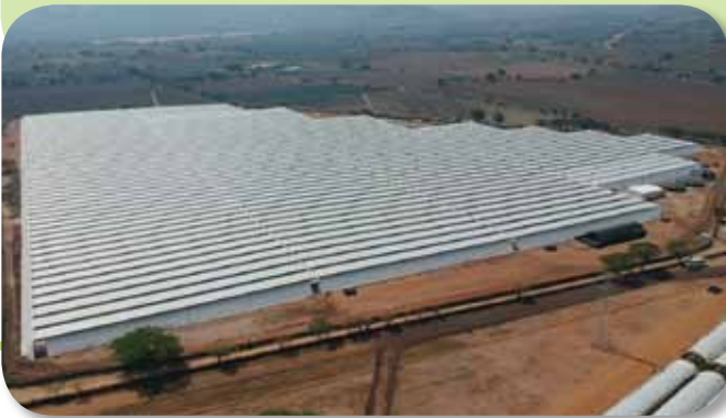
Retractable flat roof house covering 17 hectares of berries
