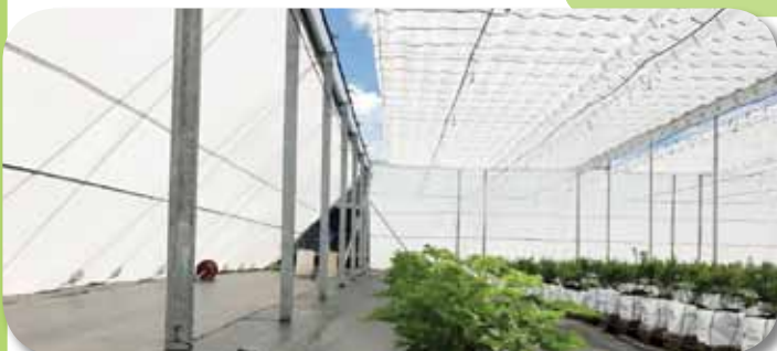
External cable bracing on all 4 walls is standard
