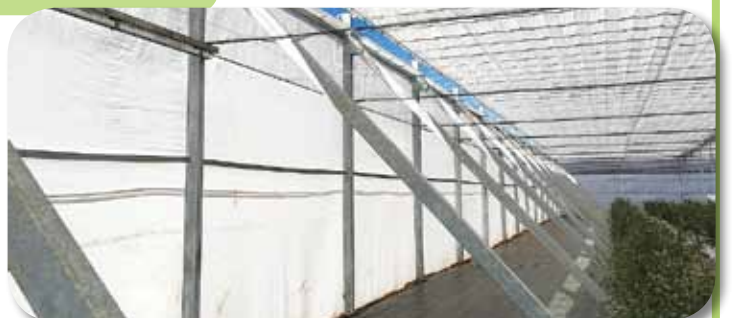
Internal interior compression bracing is an optional upgrade
